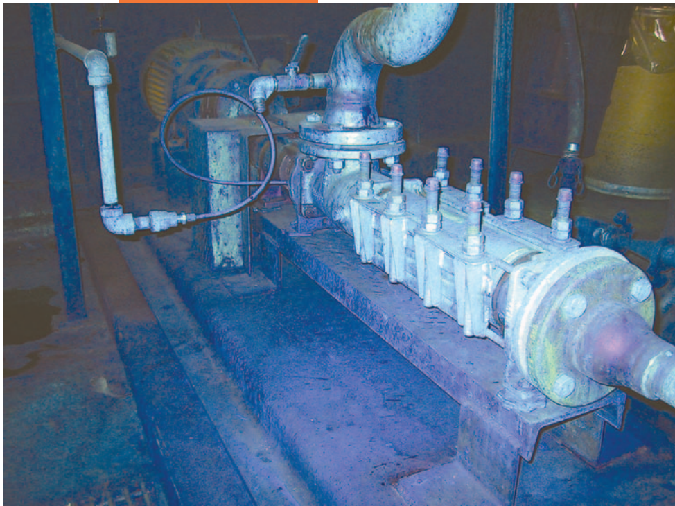
seepex's bare-shaft NS 5-12 progressive cavity (PC) pump with a molded-to-size stator outfitted with an adjustable retensioning device
